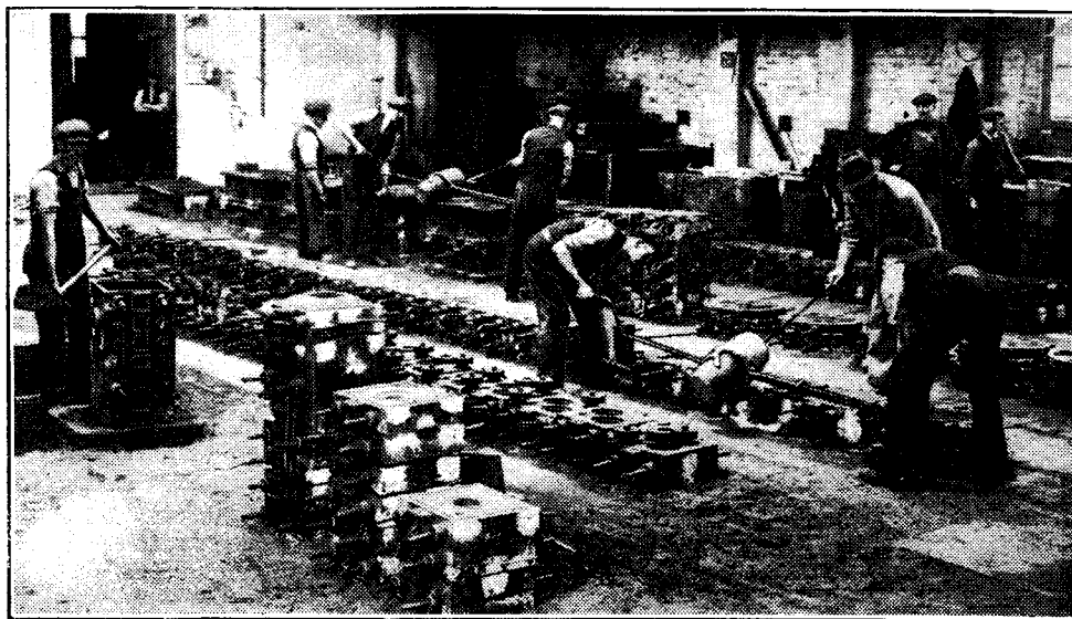
Fig. 6.—Foundry scene when making a large number of magnet castings.
