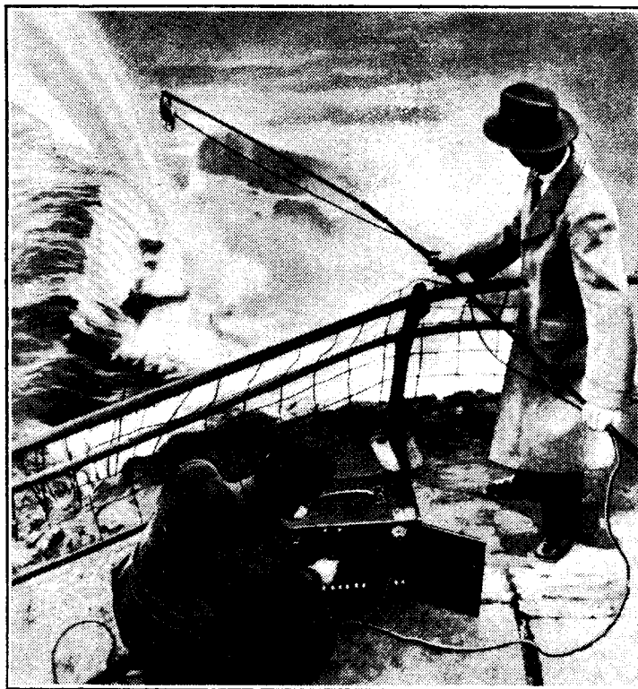
NIAGARA was a distinguished guest in a recent American network programme. Instead of relying on "effects," engineers actually went to the spot, picking up the sounds as shown and relaying them by short cable to the Niagara telegraph office.
